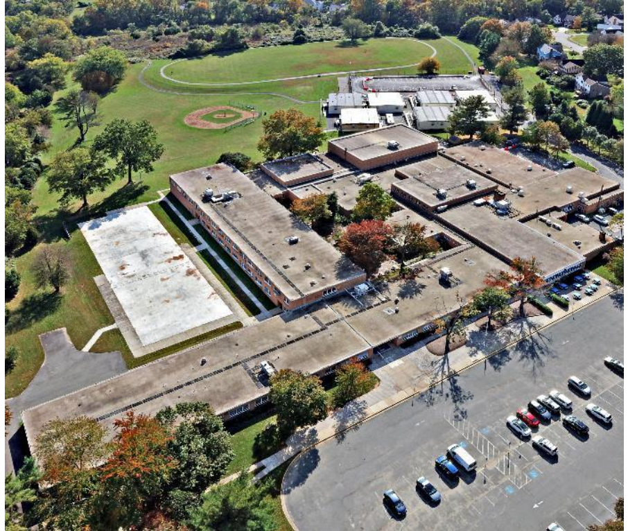
Aerial of Cooper MS with Modular Removed
