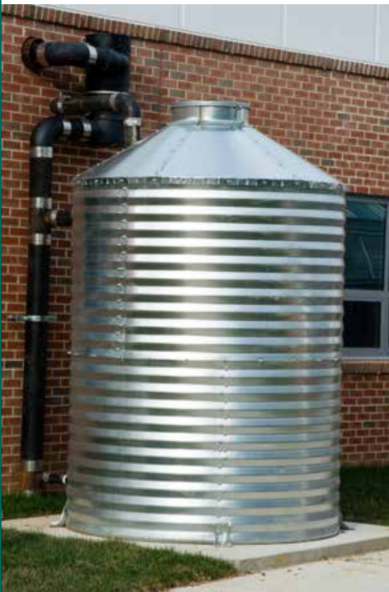
Roof rain water storage container for watering plants in the greenhouse at Thomas Jefferson High School for Science and Technology.
