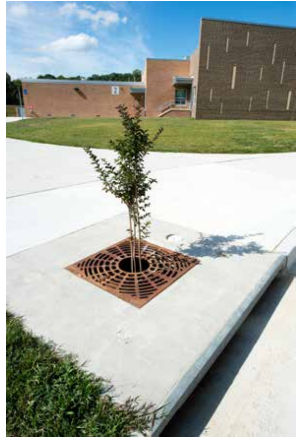
Filterras® storm water bio-filtration systems are installed to filter pollutants from stormwater at renovated schools' parking areas.
