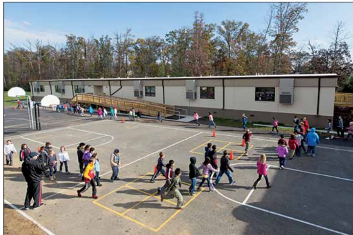
Centreville Elementary School Modular Unit
