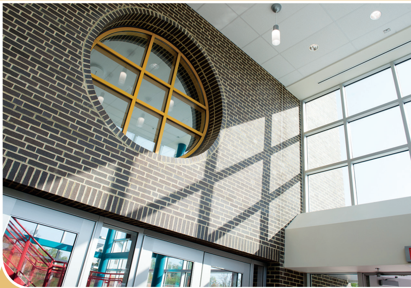
Clermont Elementary School
