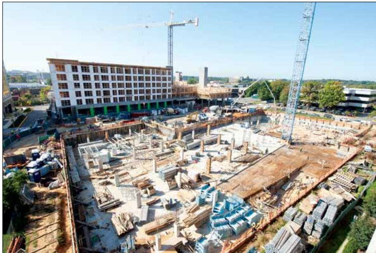
Construction in Merrifield
