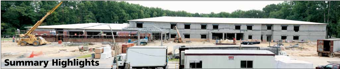
New Elementary School: Lacey Site
