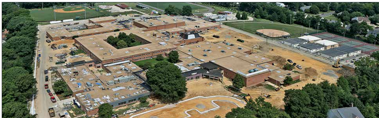
Renovations to be completed in 2014-15: Sandburg Middle School
