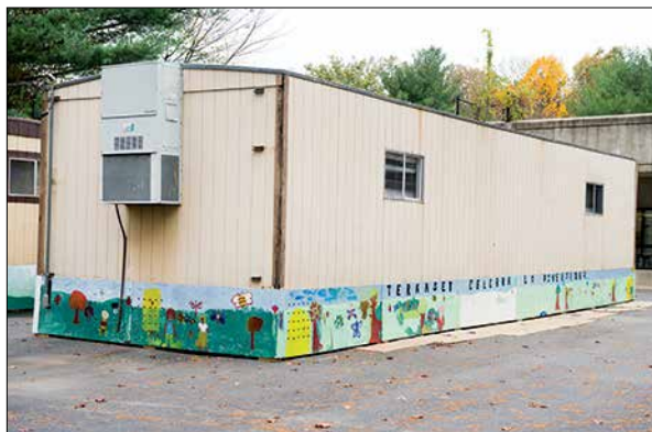
Terraset ES: Decorating temporary classrooms
