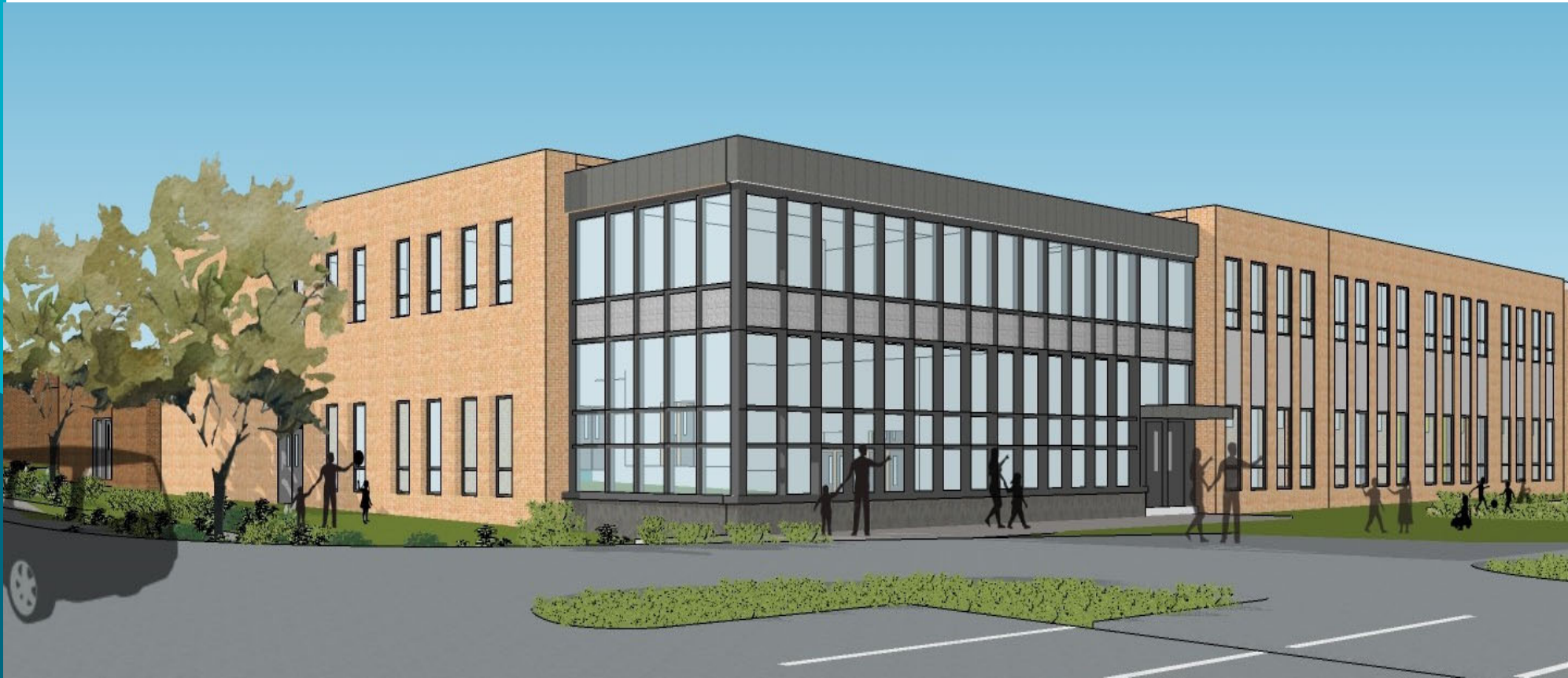
View at Cafeteria
