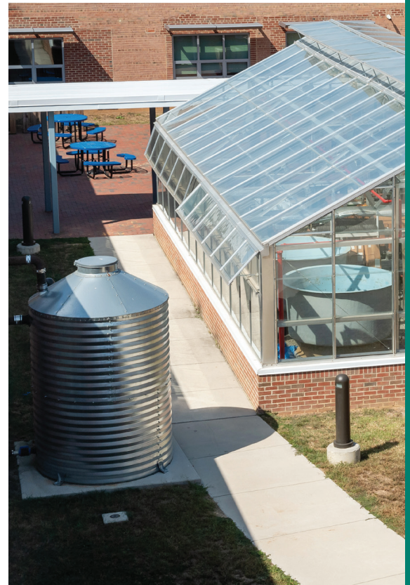
Roof rainwater storage container for watering plants in the greenhouse at Thomas Jefferson High School for Science and Technology.
